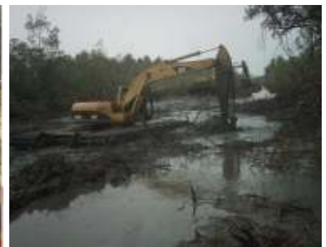
Swamp Pipeline Ditching Activities
