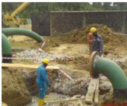
Pipeline Manifold Rehabilitation
